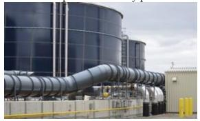
The pretreatment plant at the Bridgeton Landfill includes four, 1-million gallon storage tanks.
